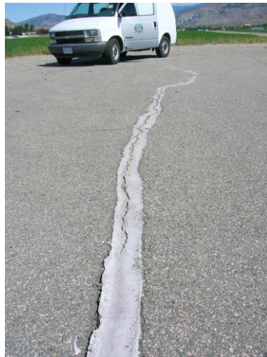
Examples of runway surface condition – open and sealed cracks
