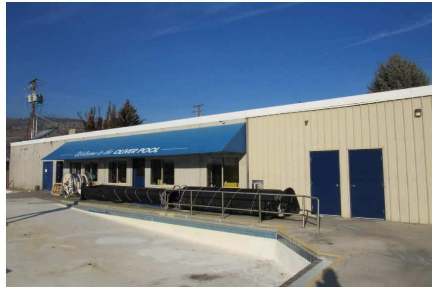
Photo #A6: Exterior cladding, windows, and utility doors at the Pool.
