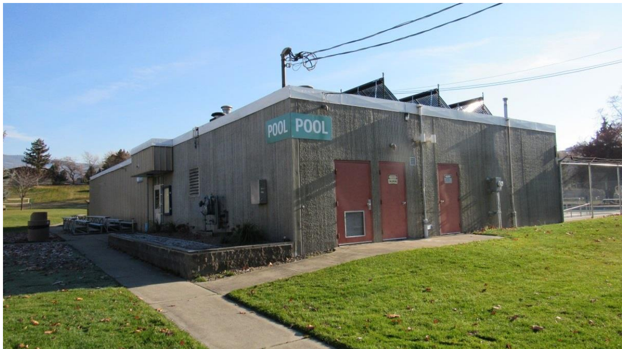
General view of the Pool building.
