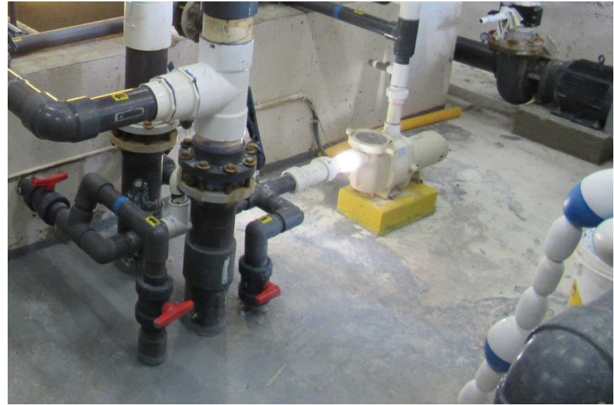
Photo #S2: CIP concrete floor slab at the Pool.
