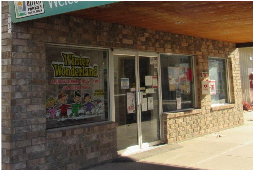
Photo #A5: Exterior entrance door and windows at the Community Centre.
