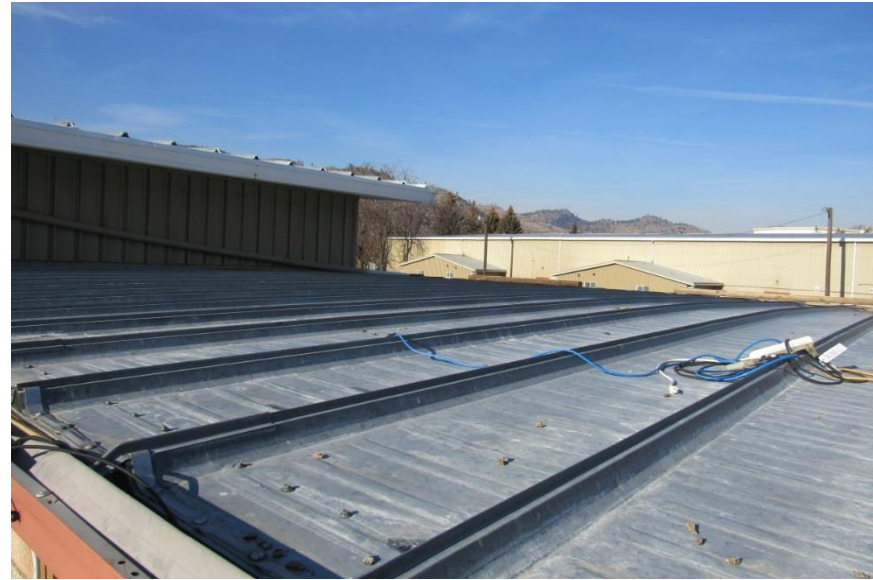
Photo #A14: Metal roof at the Community Centre.
