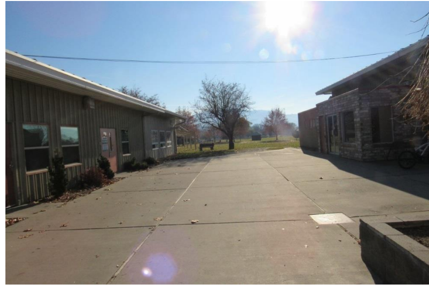
Photo #A2: Concrete walkway at the Community Centre Courtyard.
