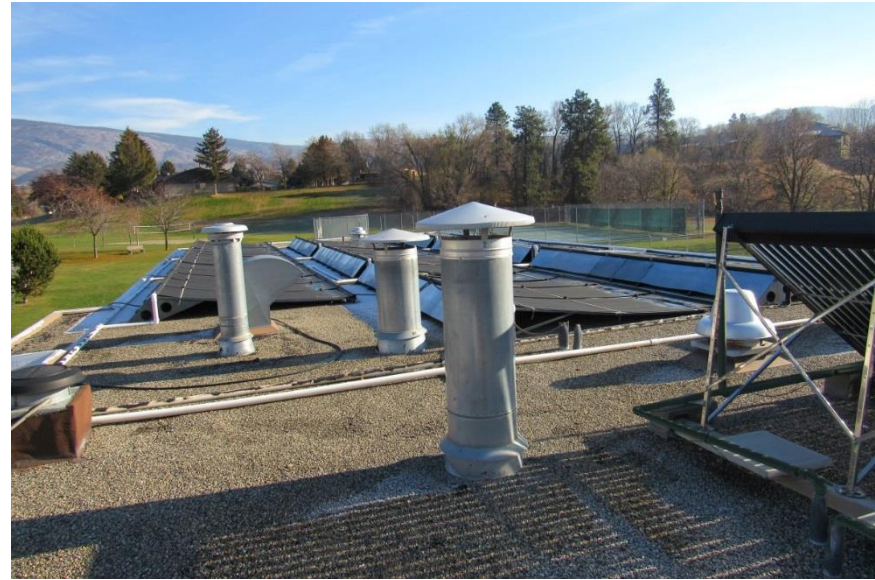
Photo #A16: Built-up roof at the Pool.
