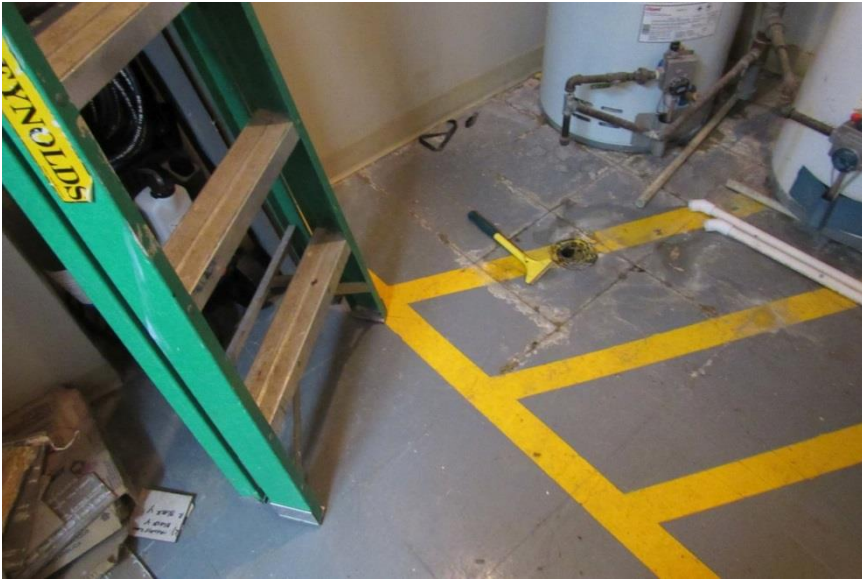
Photo #S1: CIP concrete floor slab at the Community Centre.
