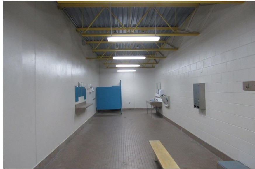
Photo #A12: Interior finishes of a Pool Change Room.
