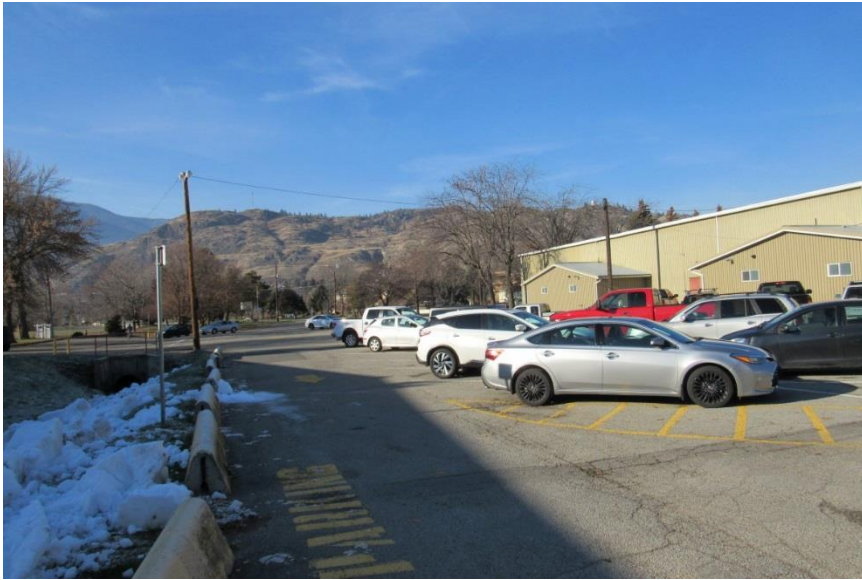
Photo #A1: General view of the asphalt parking lot.
