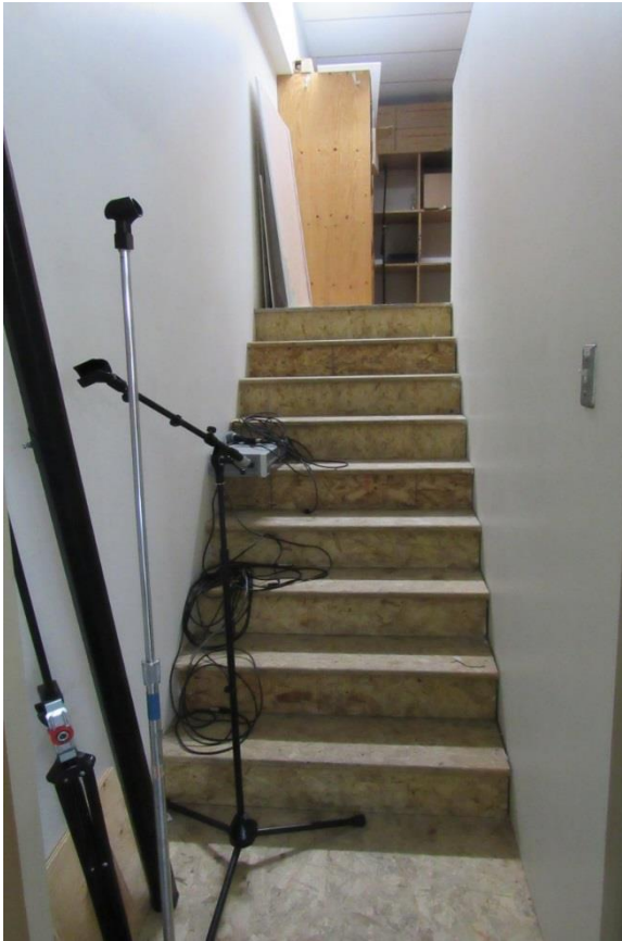
Photo #S3: Wood-framed storage mezzanine at the Community Centre.
