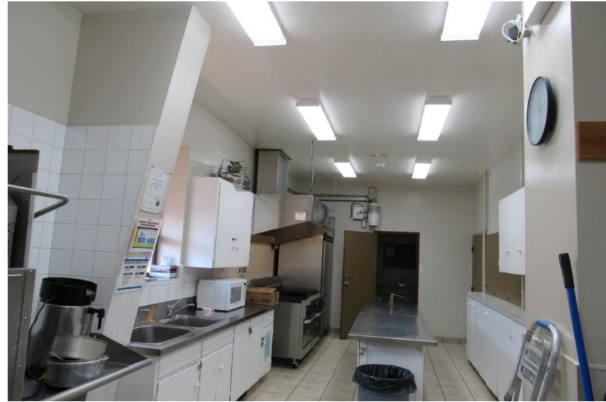
Photo #A8: Interior finishes at the Community Centre Kitchen.
