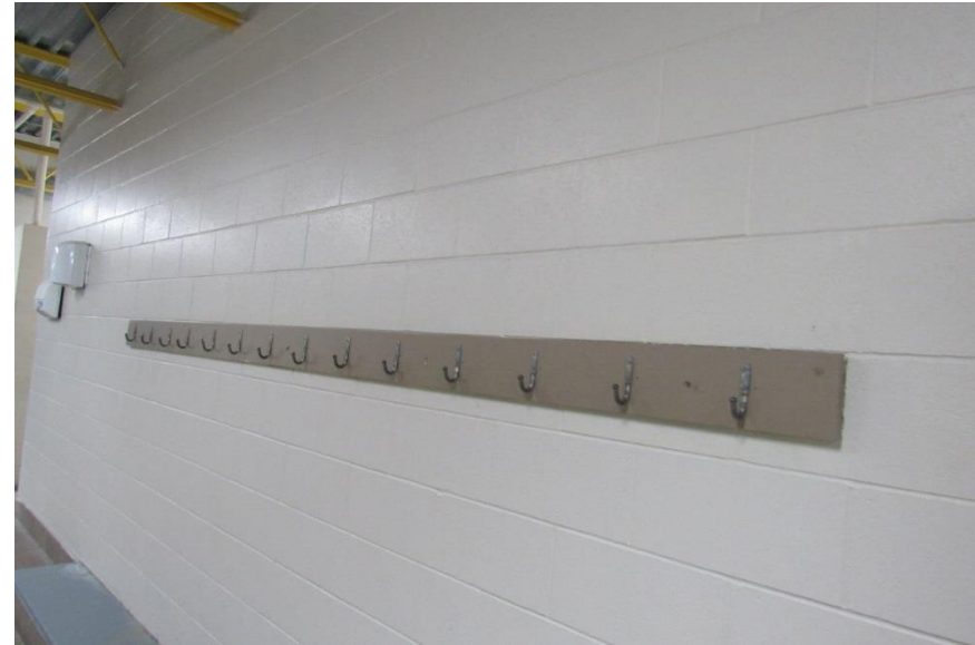
Photo #S6: CMU interior wall at the Pool building.
