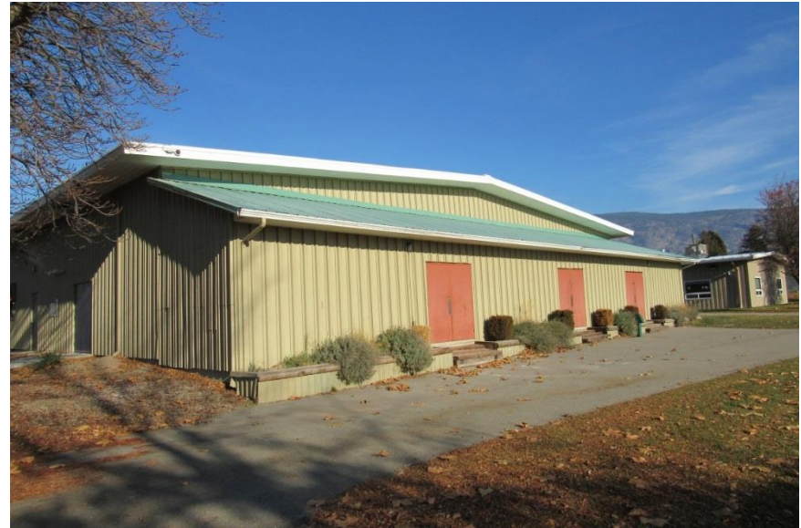
Photo #A4: Exterior cladding and utility doors of the Community Centre.
