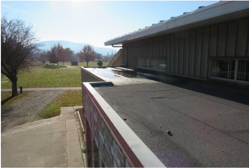
Photo #A15: Modified bitumen roof at the Community Centre.
