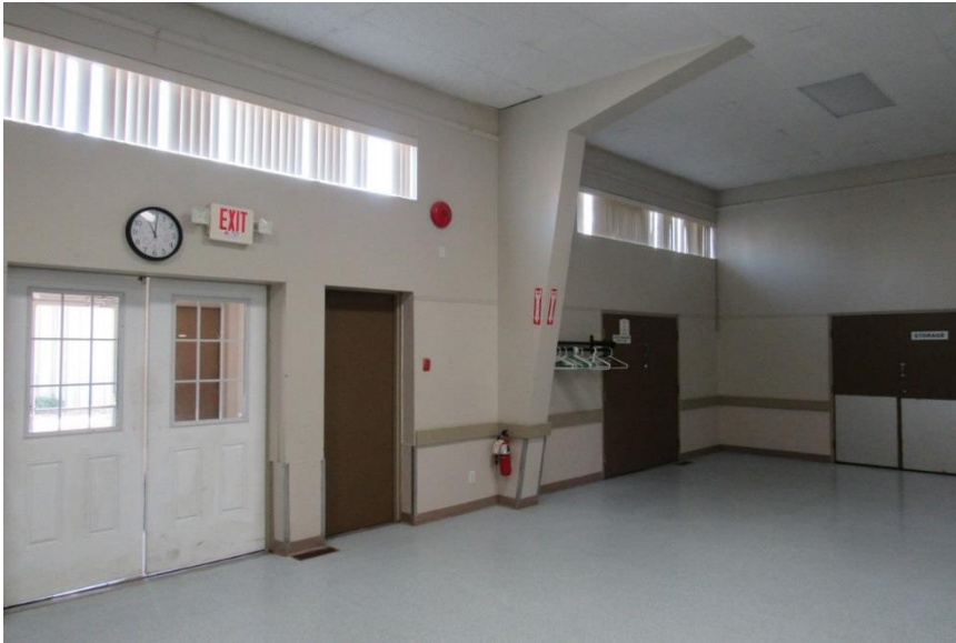
Photo #S5: Exterior wall column at the Community Centre.
