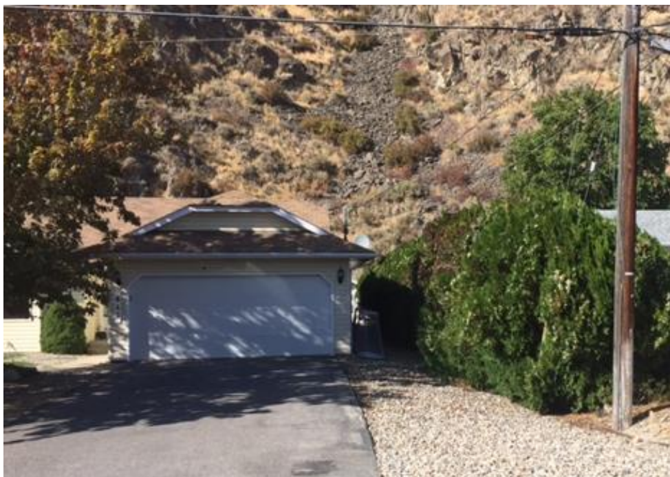
Figure 11 The choice of any particular siding material on its own does not dramatically increase the hazard rating of a structure. The presence of nearby vegetation and combustibles that can ignite with relative ease, and in turn ignite the siding or eaves, is of much more concern, as illustrated by the cedar hedge against the home in this photo.
