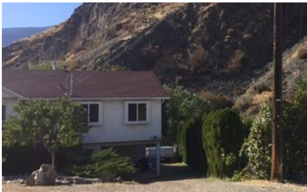
FIGURE 14 Carports should be assessed for any combustible items stored during the fire season, as this material could be receptive to embers and ignite during a wildfire. The cedar hedge is presenting a fuel hazard to this home, particularly the carport area which can act as a heat trap should the hedge ignite during a wildfire.
